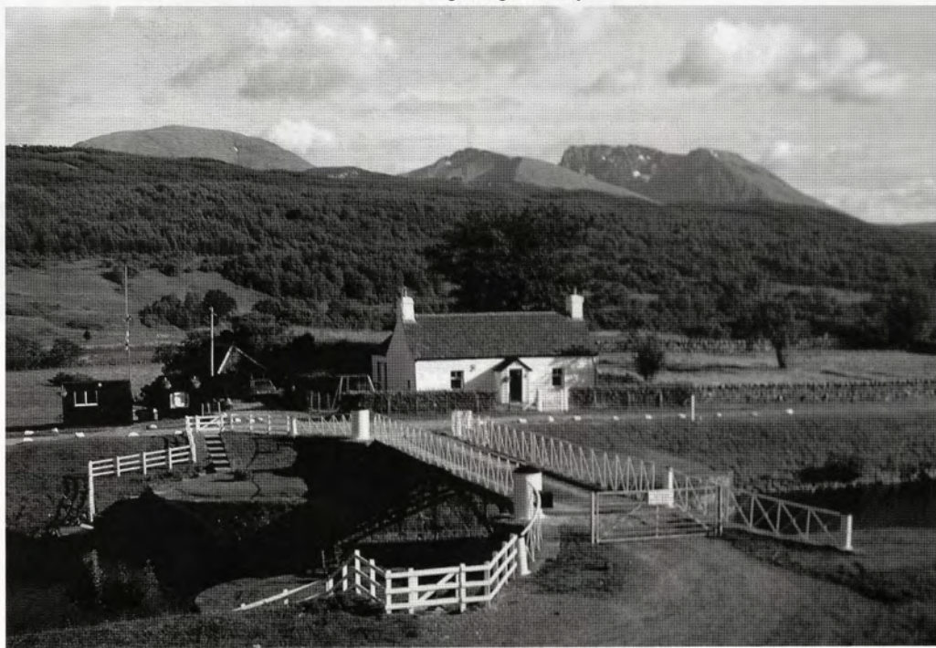
Canal swing bridge at Moy
