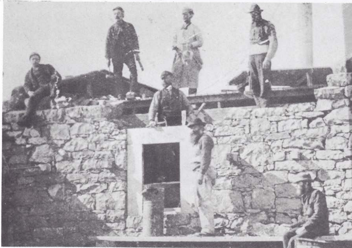
Construction work on the Ben Nevis Observatory which was completed in 1883.
