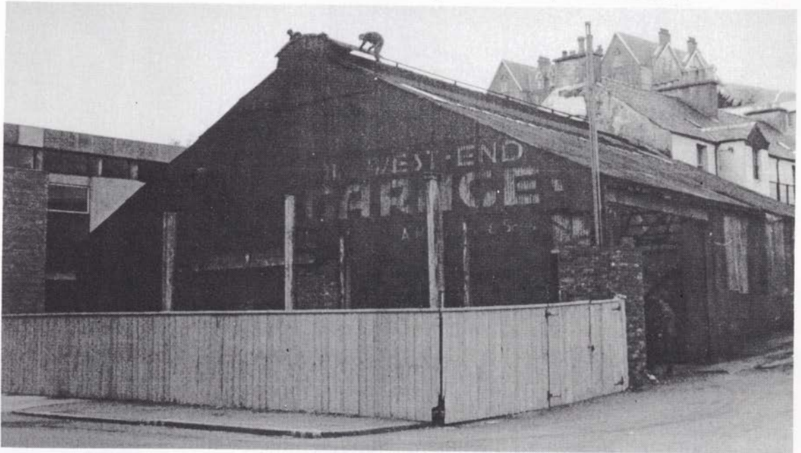
The same site as above: Macintyre's West End Garage in the process of demolition C. 1963.
