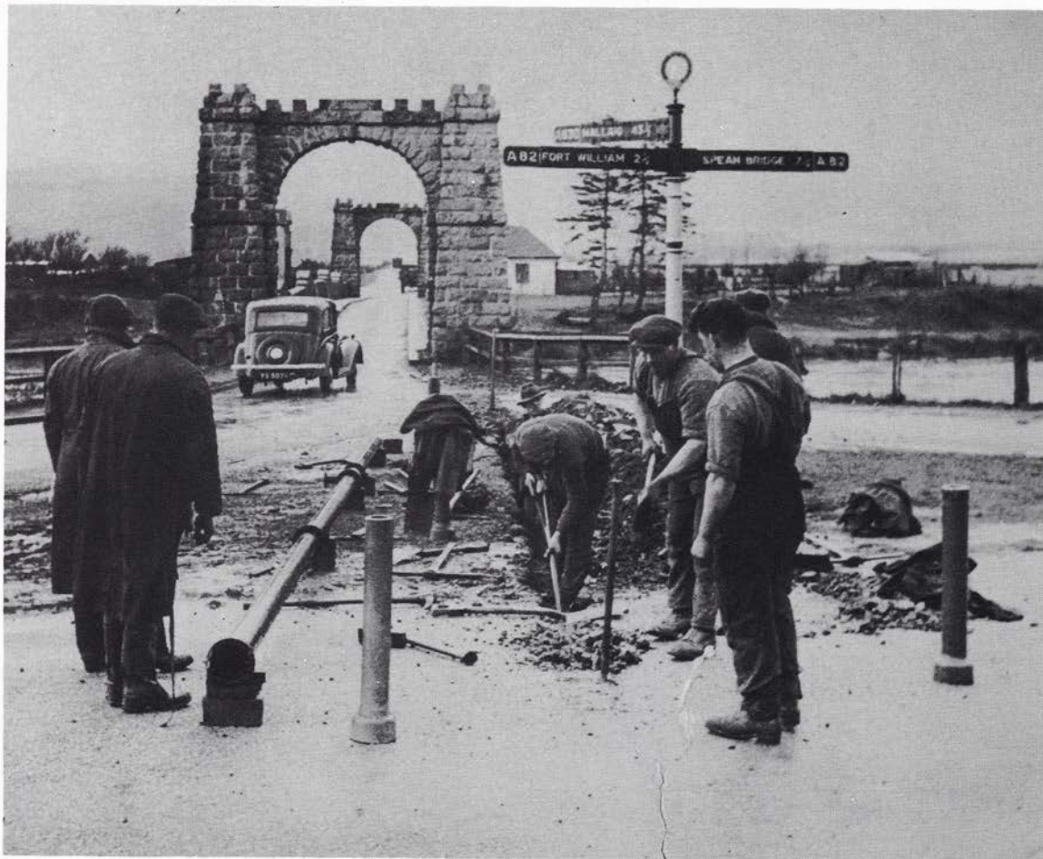
Pipe laying at Lochy Bridge in the fifties.
